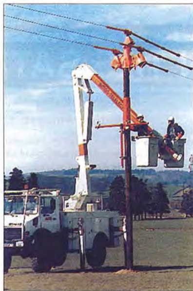
The "insulating aerial device" allows linesmen to carry out work on the poles.
