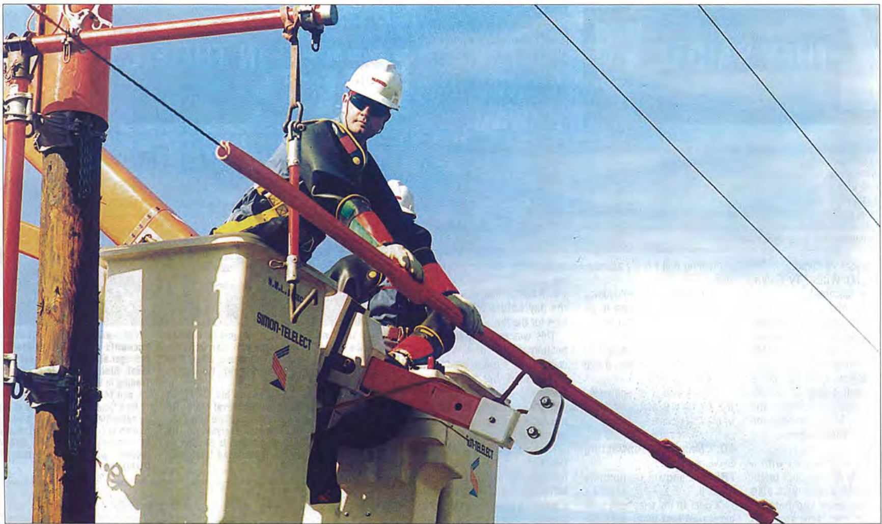
Live line workers applying protective shrouding to conductors.
